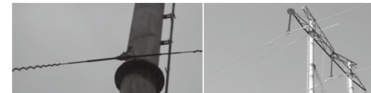
Installation on pole
